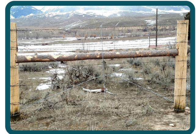
**Corner brace:** Any brace at the corner of a fence.
